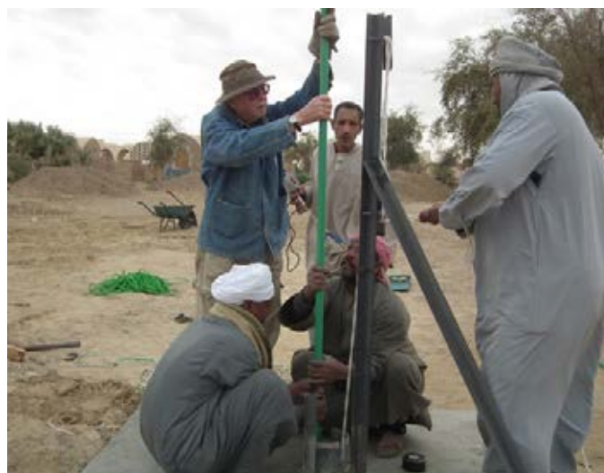
All hands on deck: Joe lowering the pump into the well.
