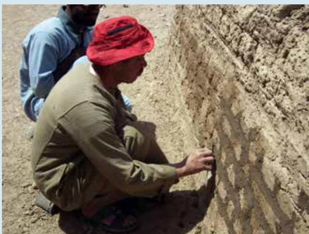
Touching up the mud grout on the perimeter wall.
