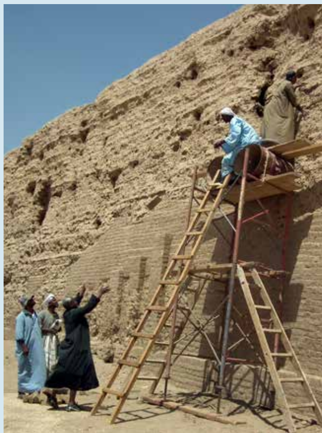
Tip-top repair work!
