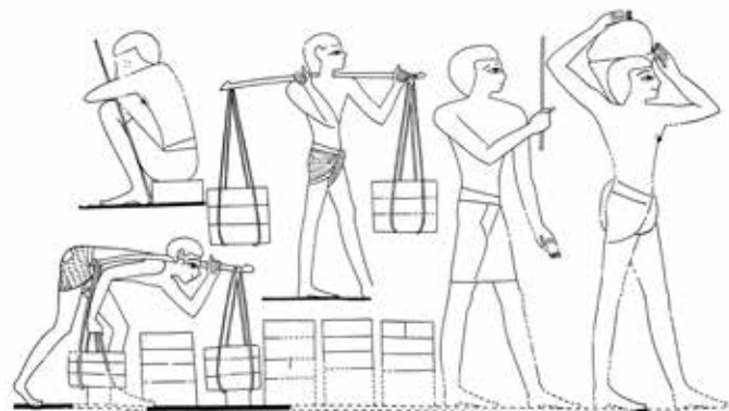
Transporting bricks and materials. Scenes from the work site in the Tomb of Rekhmire, 18th Dynasty (after Davies 1935: pl. 59).
