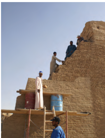
Nearing the top in the northeast.
