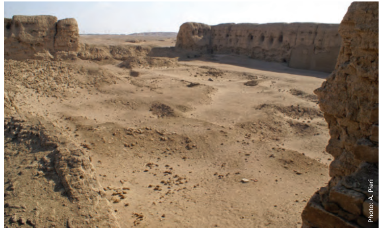
Interior view from 8 meters up!
