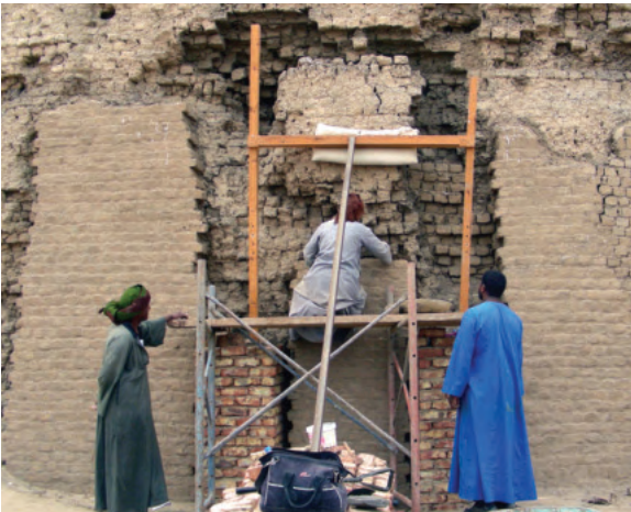
Final fixes on the Fort interior.
