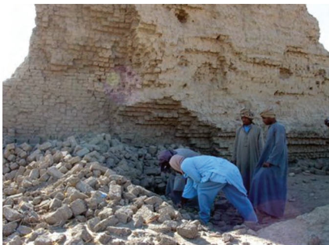
Collapse at the northeast corner — the event that started it all off.
