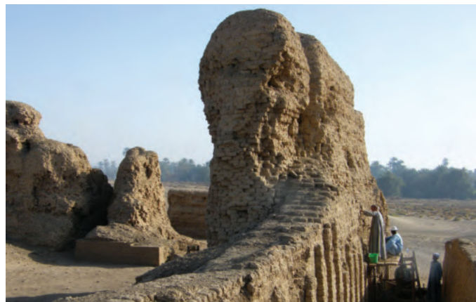
Shifting fortunes: the south wall segment is leaning inward. Help!
