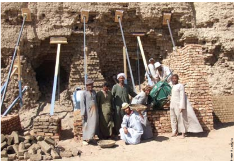
The dedicated crew applying the final touches to the temporary supports.
