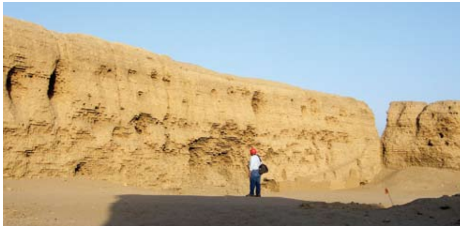
Richard contemplates the crumbling central gap.
