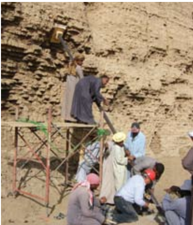
Emergency repairs underway.
