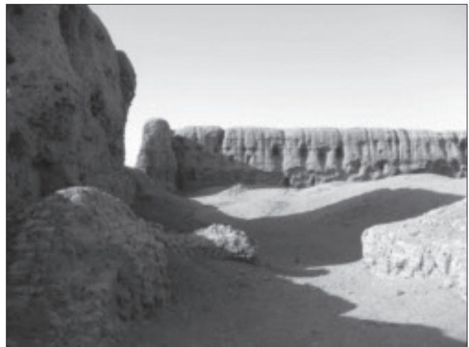
The Fort: now it's an inside job...
