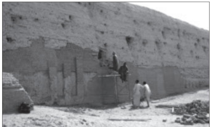
The ugly central gap before (above) and after (below). It's history!
