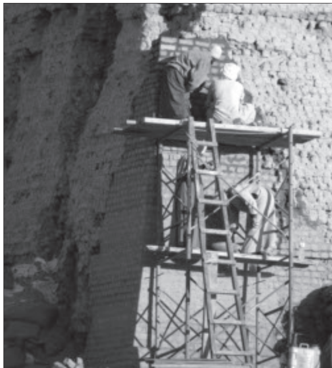
Mission accomplished: finishing up at the southwest corner.
