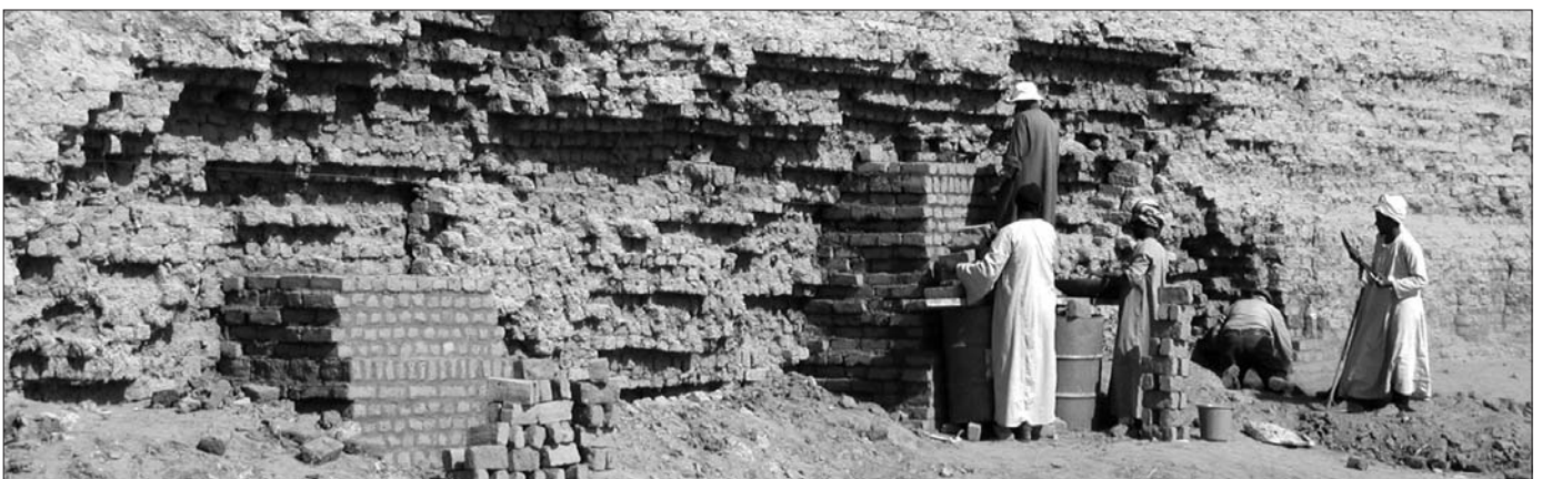
Building the buttresses in the "central gap."
