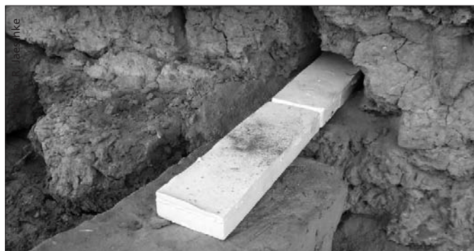
Plaster bar inserted to monitor movement.
