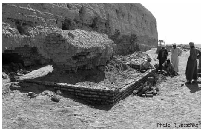
Building the brick box around the perimeter wall.
