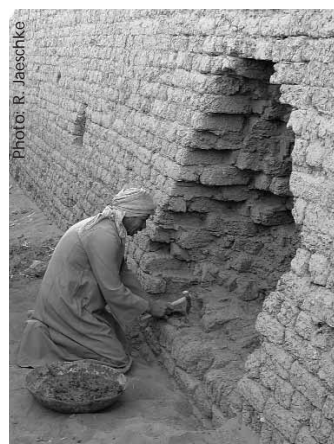
Abdullah preparing the hole in the south wall for repair.
