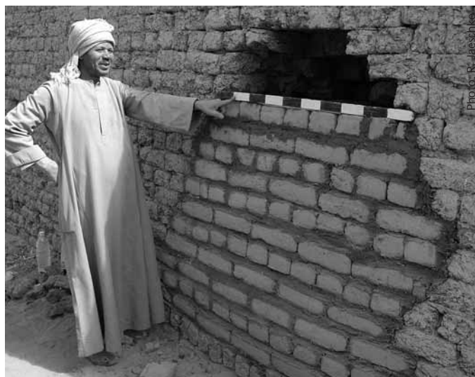
Filling the breach with new bricks following the ancient pattern.
