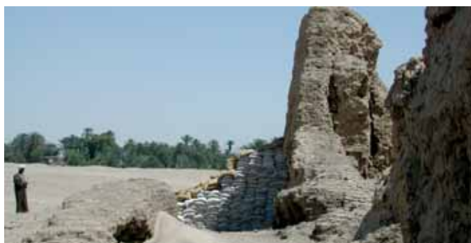
Sand bags at the corners provide temporary support.
