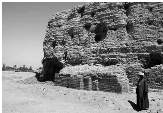
The perimeter wall repaired.
