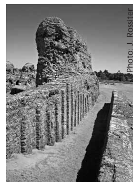
Pilasters along the south wall.
