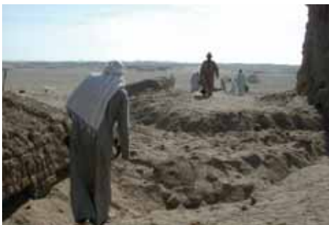
Bringing in the dirt to raise the lower ground level by over 1.5m.
