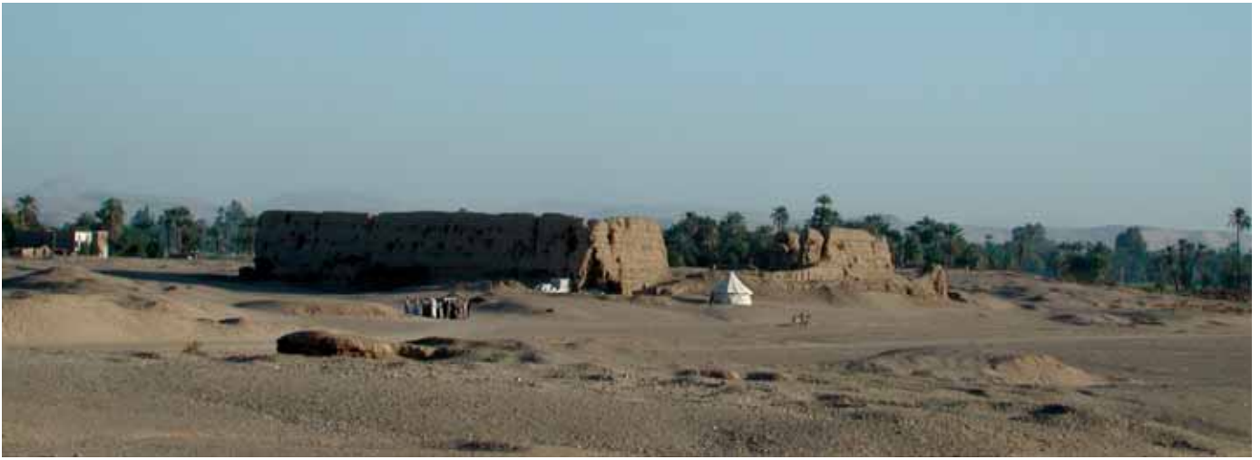
Repairing the Fort....see page 24.
