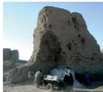
Sand bag delivery to the precarious Northeast corner.
