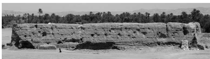
The west wall in March 2005 after repairs.
