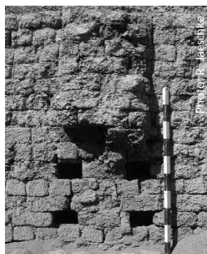
The pilaster during repair.
