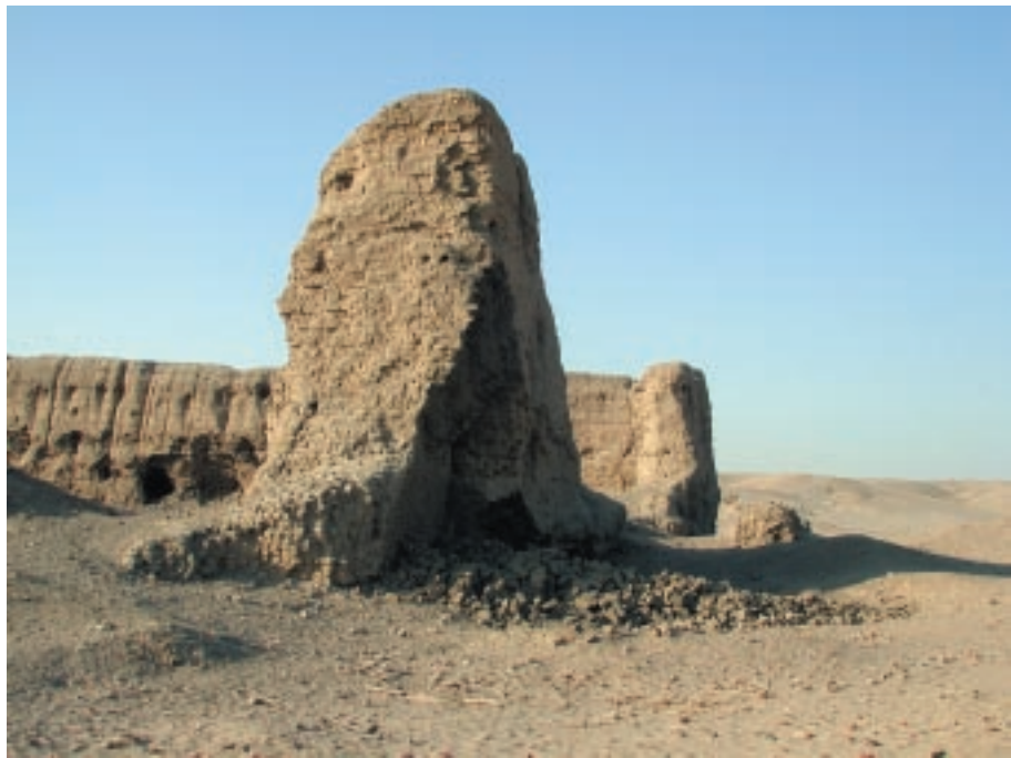
The Fort falls down; the recent collapse of the NE corner.
