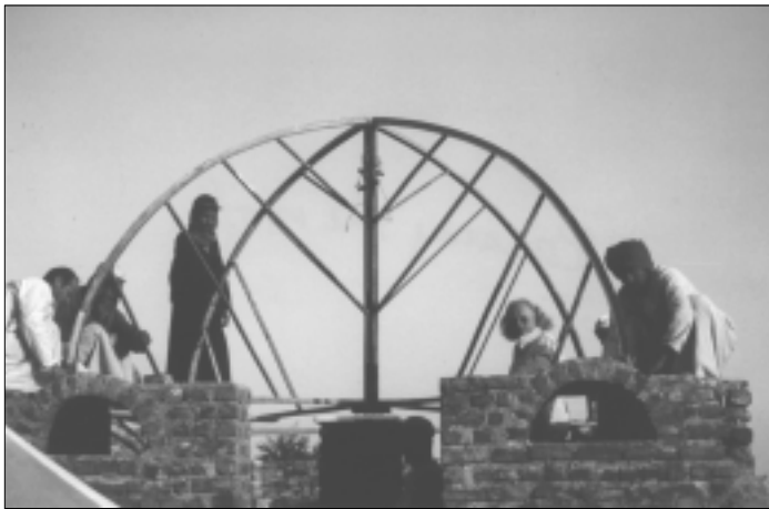
Günter Heindl helps raise the roof over more new rooms.
